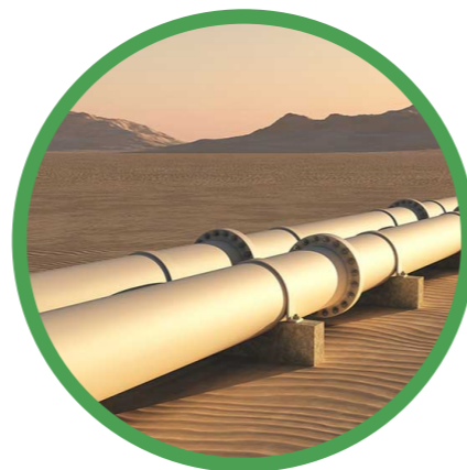
PIPELINES AND TANKS
